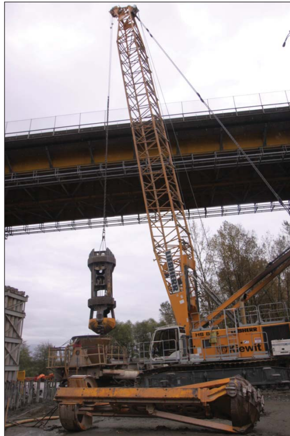
Figure 1.5 - An oscillator is necessary for the drilled shafts operation.
