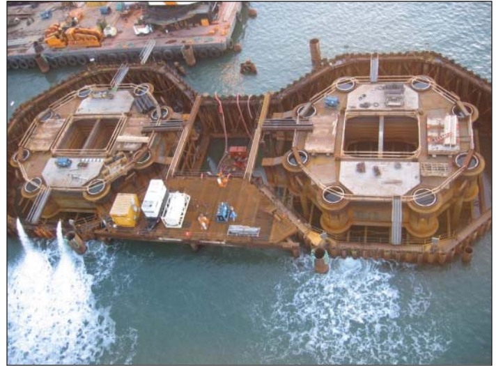
Figure 1.4 - Cofferdam is a structure used to isolate a work area from a water body.
