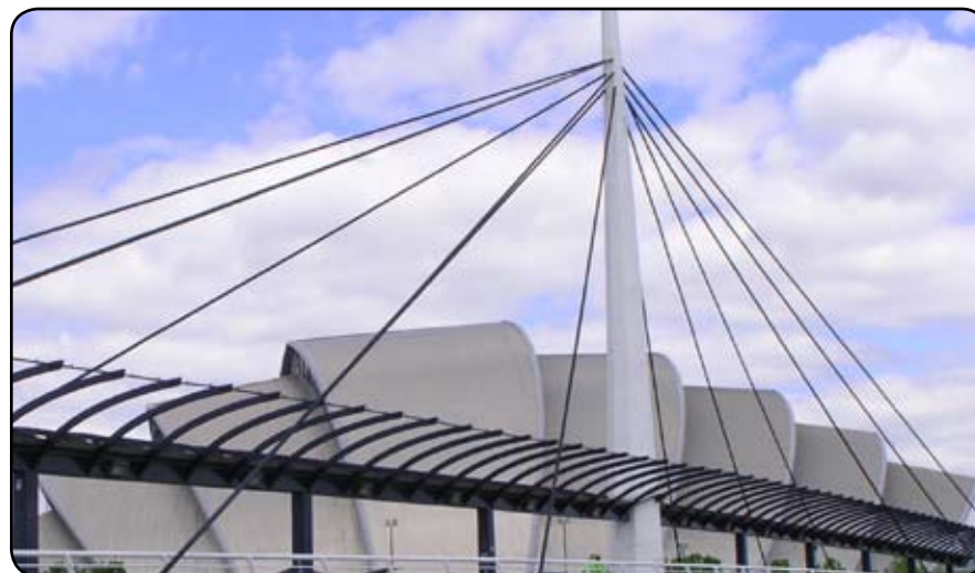
Example of a fan design. Image used under a Creative Commons license. Source: flickr.com/photos/limowreck666/146131114/
