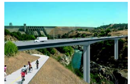
Folsom Dam Bridge, Folsom, CA
