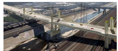
6th Street Viaduct Bridge, Los Angeles, CA
