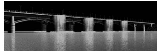
Cypress River Bridge, Sacramento River, CA
