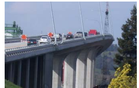
Maxwell Replacement Bridge, Napa, CA
