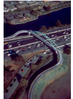
I-80 Bicycle/Pedestrian Overpass, Berkeley, CA
