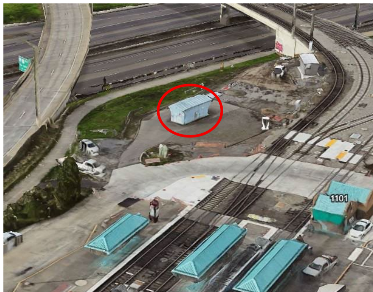
Traction Power Substation, Gateway/NE 99th Ave Transit Center
