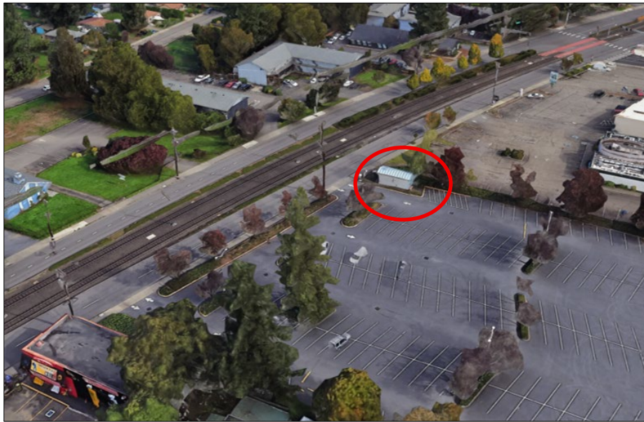
Traction Power Substation, E 181st Ave Park & Ride
